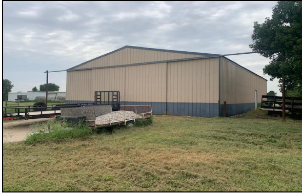
East View of Machine Shed Door Open for 40' Entrance
